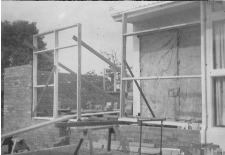
Figure 18: Lavery House second stage under construction, nd (c. 1955). Eastern addition to the house wing. Original Bedroom and Living area window walls re-used in the addition. (Source: Lavery Family courtesy of Piers Lavery, October 2020)
